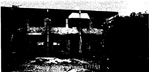
AWAITING COMPLETION - THE UNFINISHED FACULTY HOUSING PROJECT - JANUARY 2001
